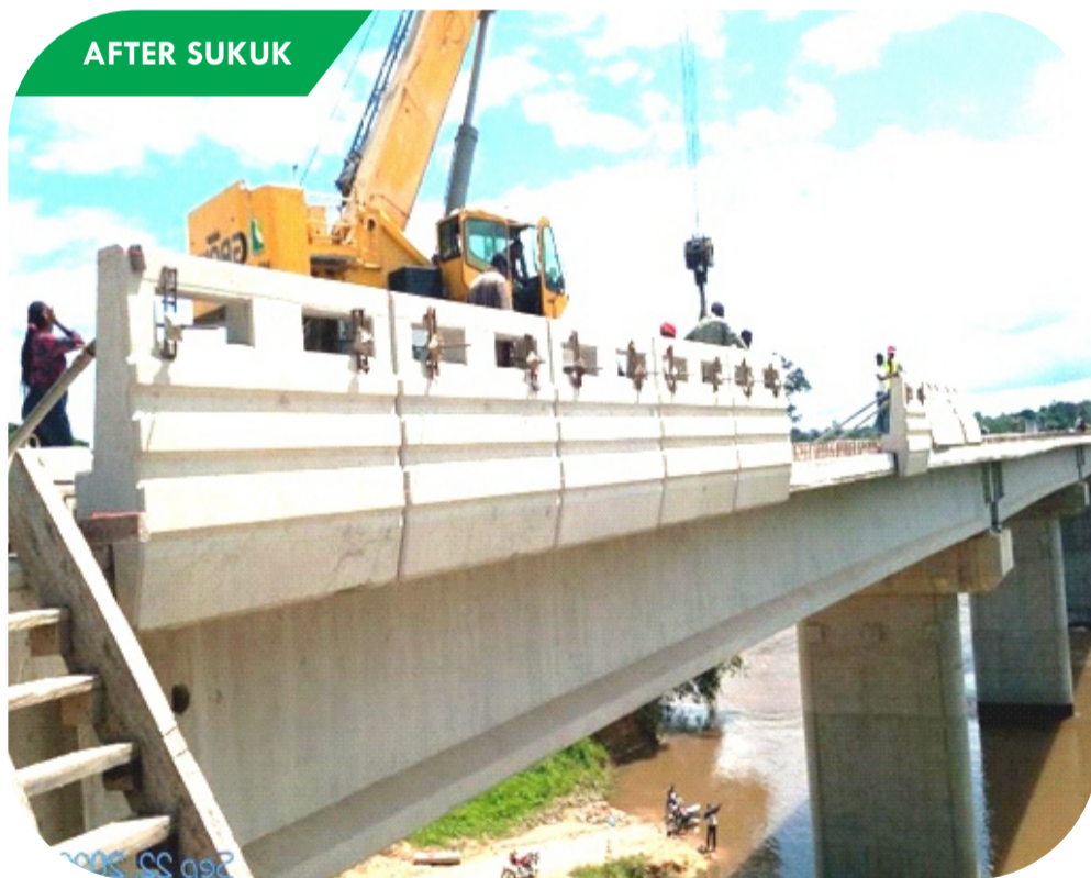
CONSTRUCTION OF IKOM BRIDGE IN CROSS RIVER STATE
